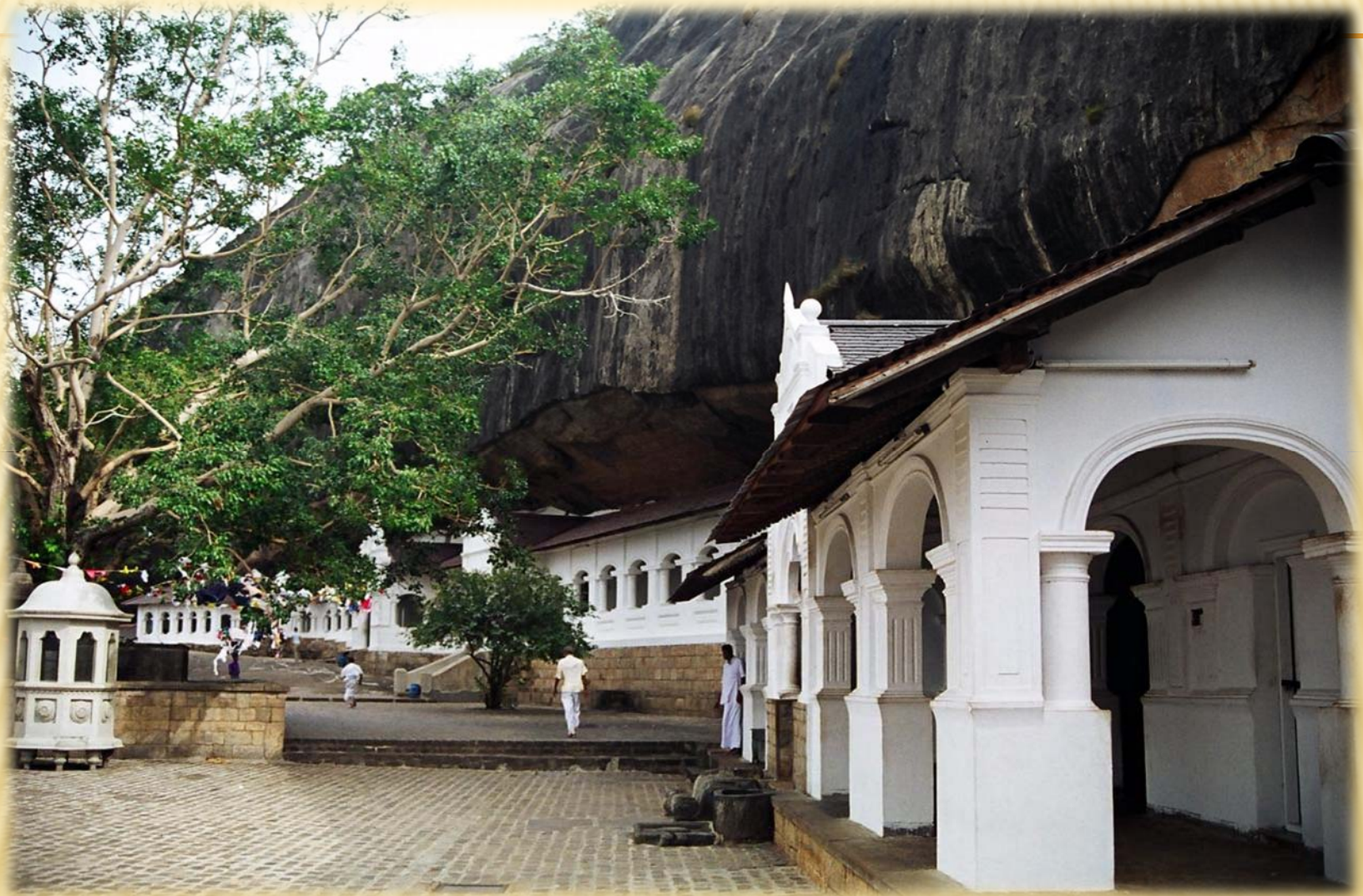
The facades that protect the cave interiors. You can see the drip ledges above.
